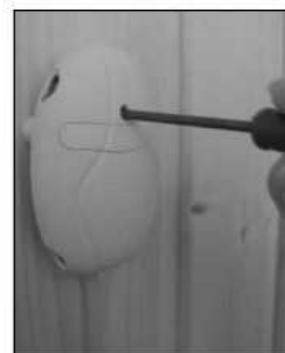
Figure 11. Reset button for overheating limiter
